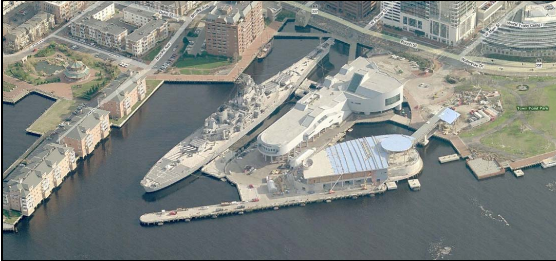
FIGURE 4: AERIAL OF HALF MOONE CRUISE TERMINAL
